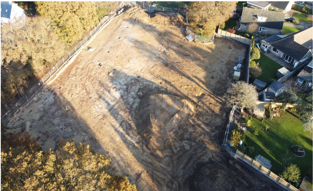
Plate 22: Aerial photo of Area 1.3, looking east-north-east.
